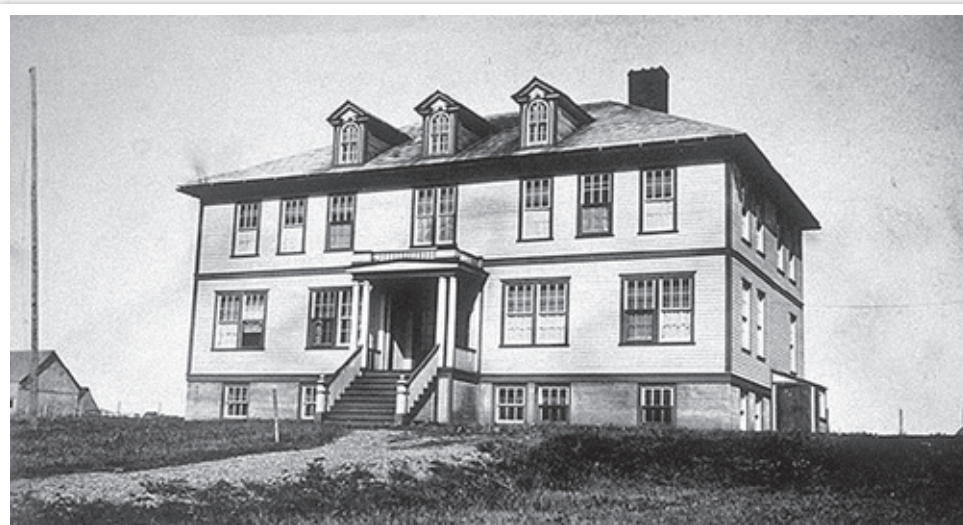
FIGURE 8 THE NEW CARLISLE SCHOOL HOME
